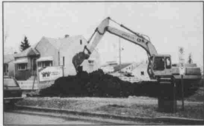
Ground is broken for Habitat's new McCauley duplex.
