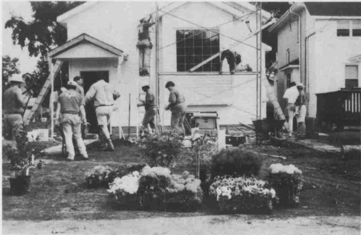
Habitat For Humanity volunteers work to build a new complex.
