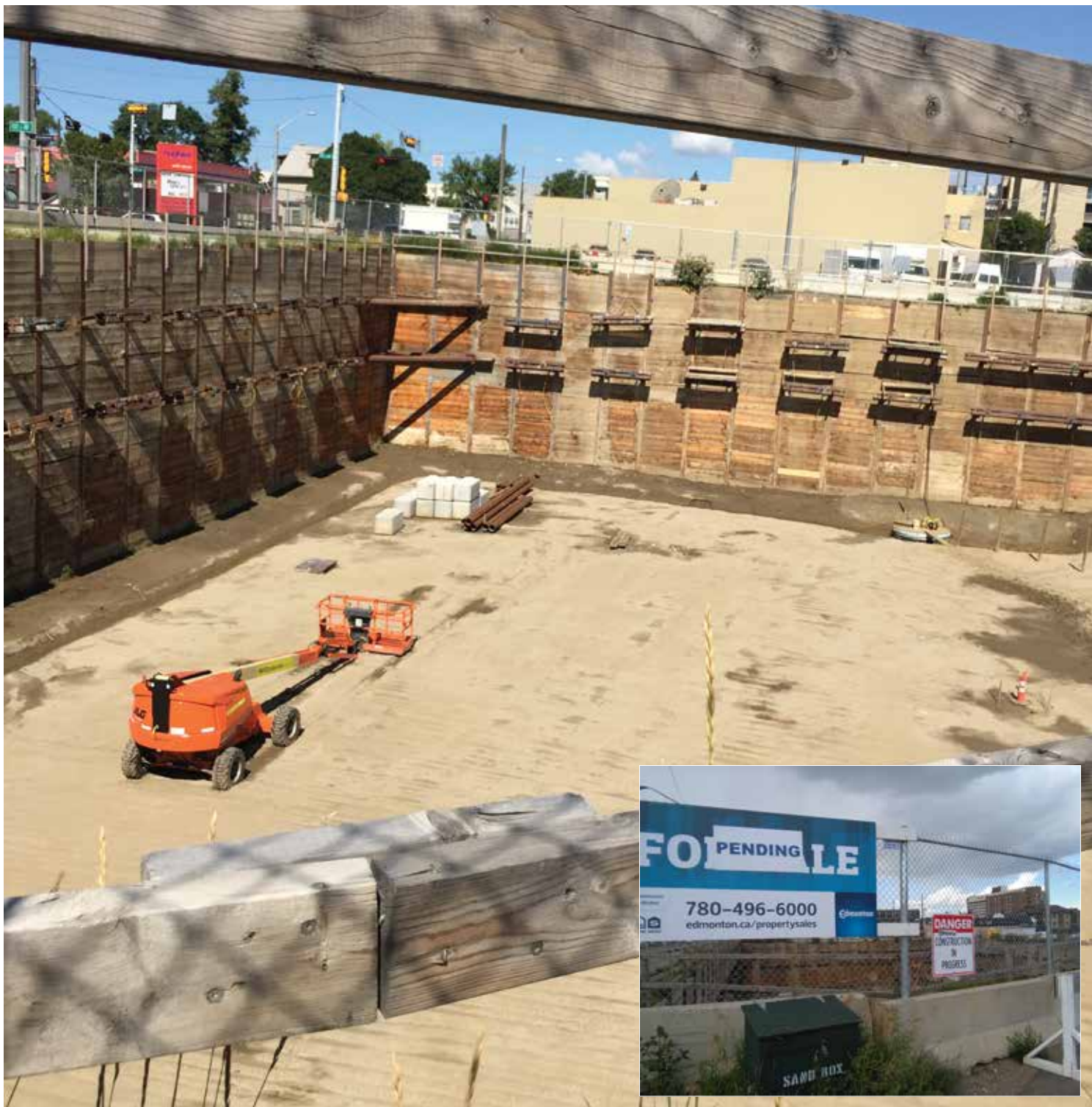
A look inside “The Hole.” Inset: signage indicating a pending sale. Dan Glugosh & Jayne Russell
