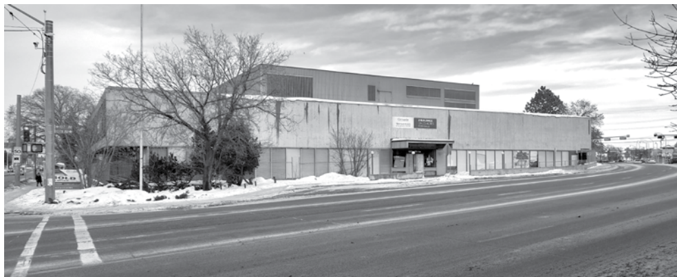
BSCS will be moving into this building at 10010 107A Avenue after it is renovated. Leif Gregersen
