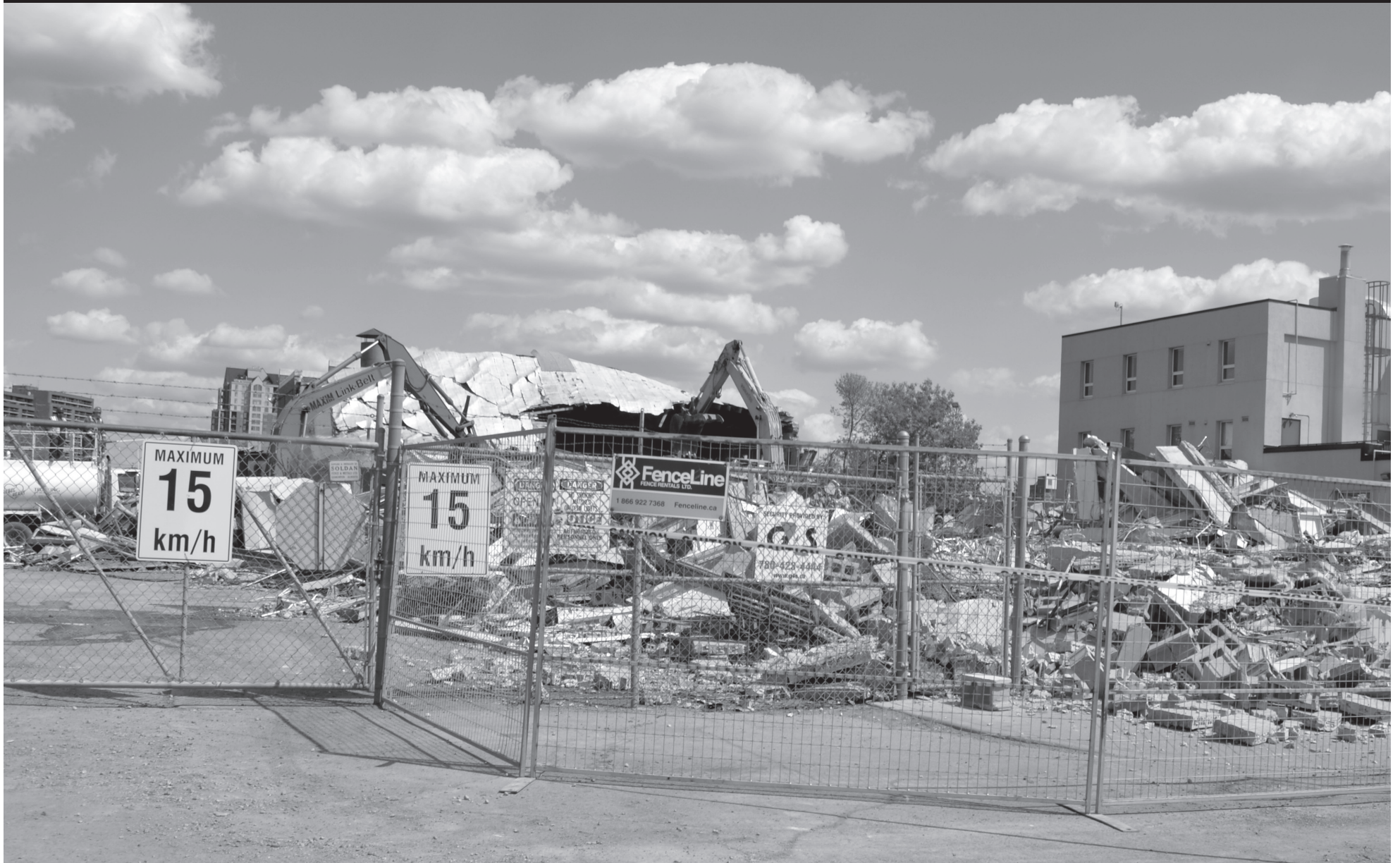
Warehouses formerly located north of Bissell Centre East on 105 Avenue and 96 Street were demolished in May to make room for the new main Edmonton branch of Canada Post. Currently located at 101 Avenue and 102 Street, it is slated for demolition to make way for the new Royal Alberta Museum. Paula E. Kirman
